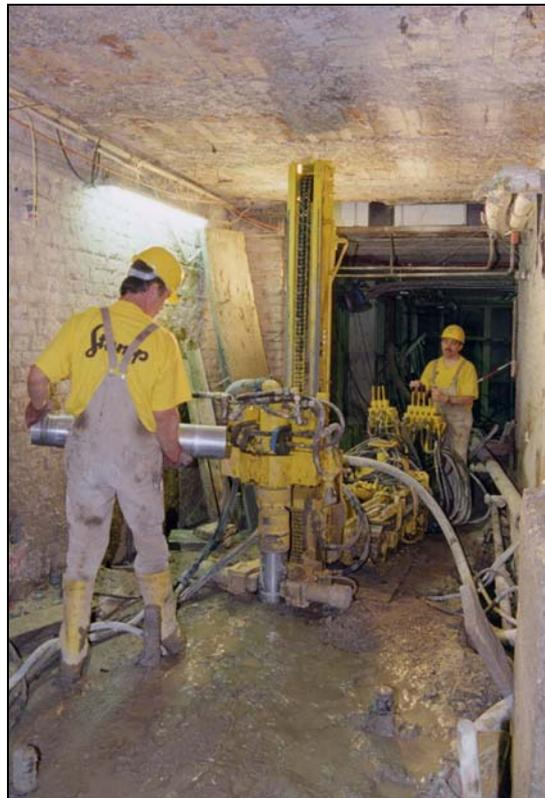
**FIG. 6:** Drilling operations for pile manufacture
